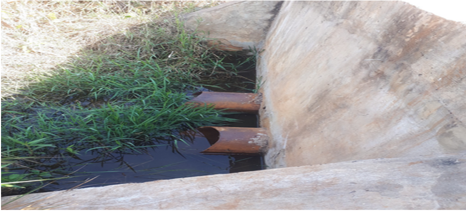
Plate 10: Rusty outlet pipes
