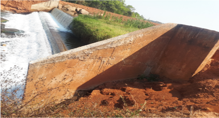
Plate 13: Erosion on the third side of the 3 rd drop structure
