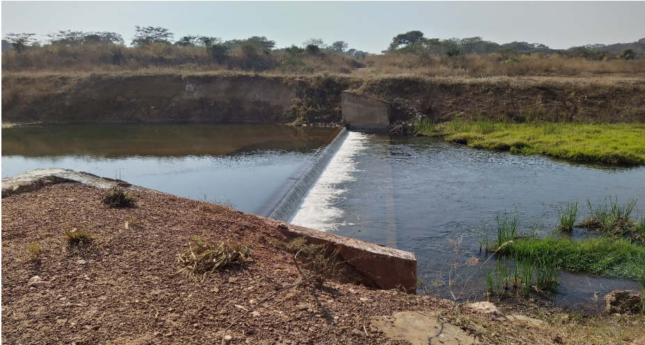
Plate 22: Spillway site showing erosion of the training walls
