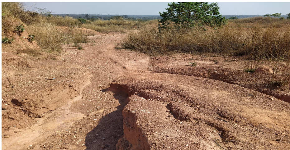
Plate 20: Access road from borrow pit to project area eroding
