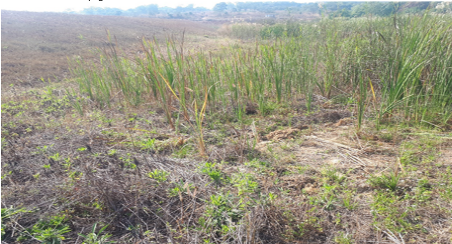
Plate 8: Presence of a soft toe on the right bank flank of the embankment
