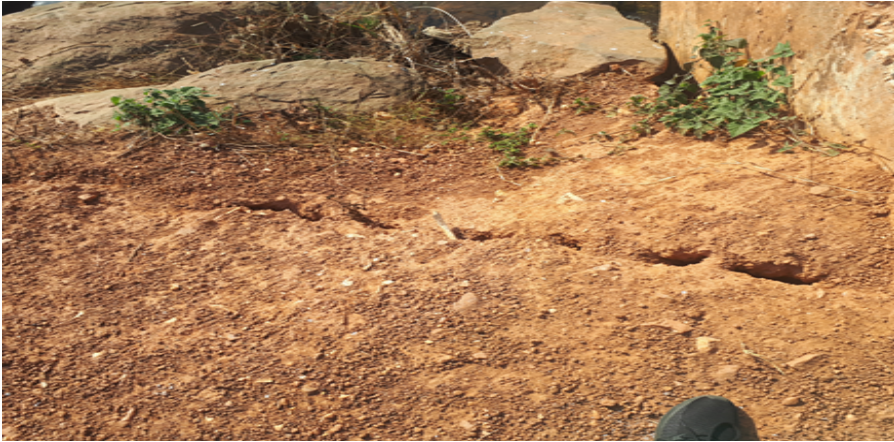
Plate 17: Crack along the training wall near the right abutment of the 3 rd drop structure
