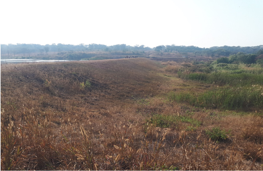
Plate 7: Downstream slope with marsh areas
