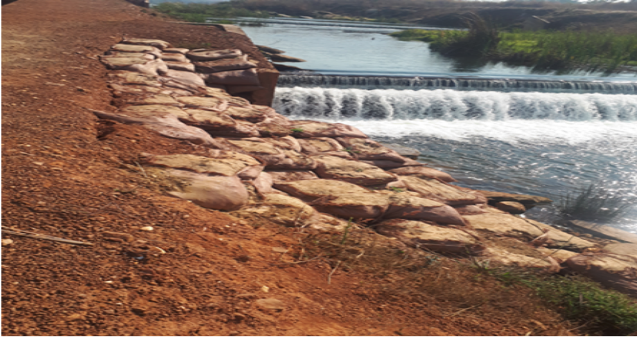
Plate 15: Erosion on the abutment of the 2 nd drop structure
