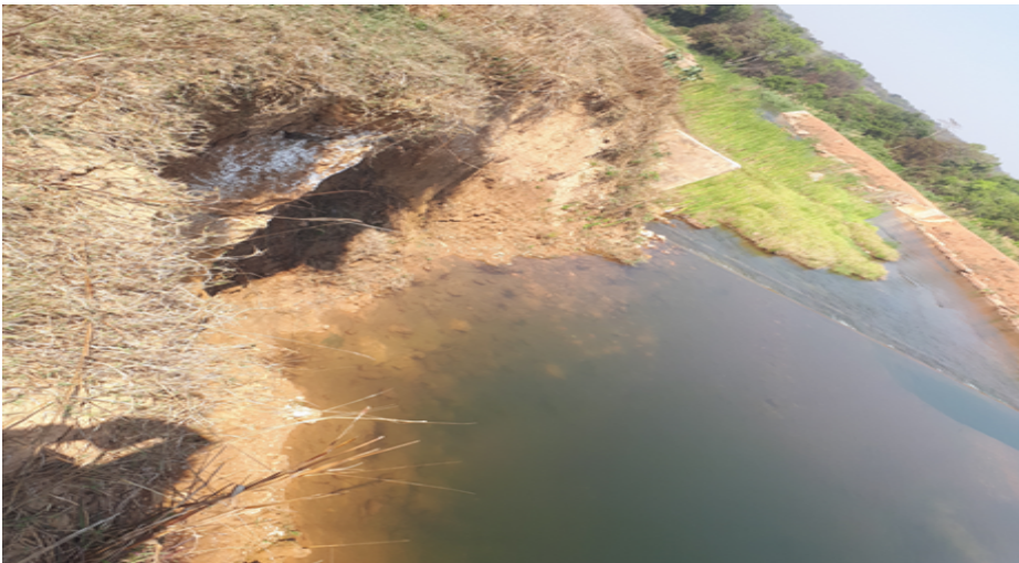
Plate 14: Erosion near the left side of the 1 st abutment structure
