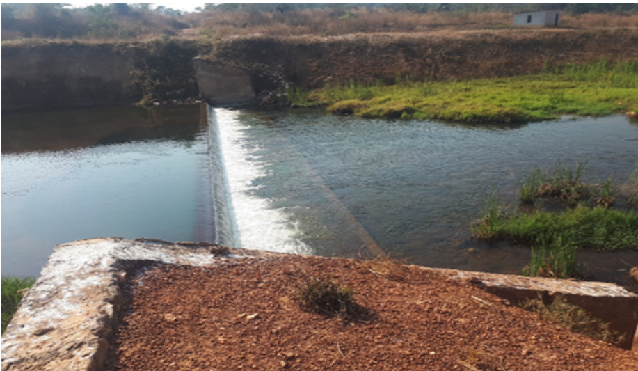
Plate 11: Incomplete emergency spillway
